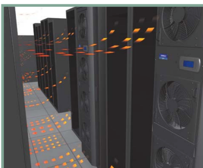
Direct rack cooling
